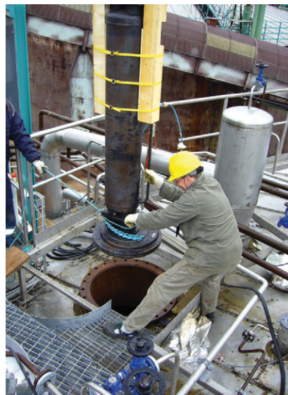
Figure 6. The manhole situated on top of the tank.
