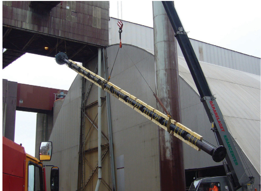
Figure 5. Bringing the pump into a vertical position.
