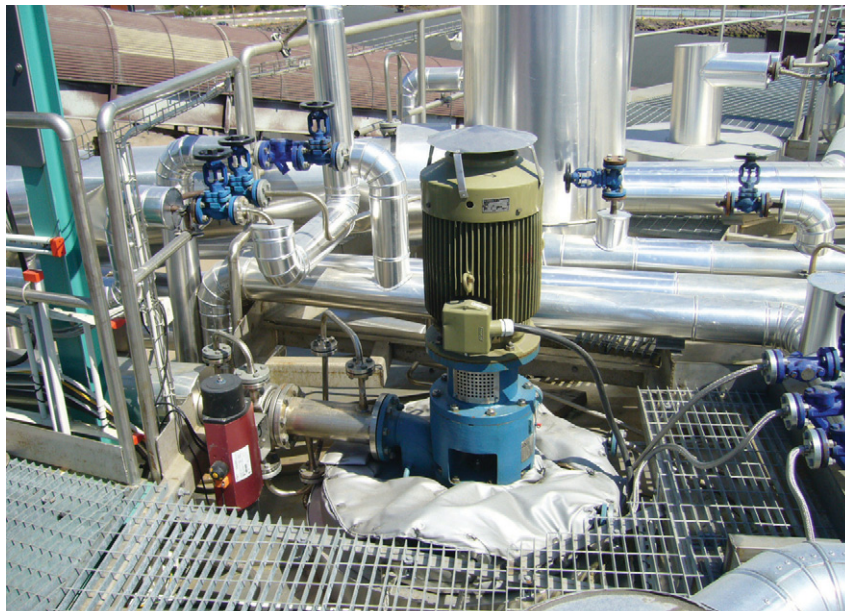
Figure 9. The installed pump at the terminal site.
