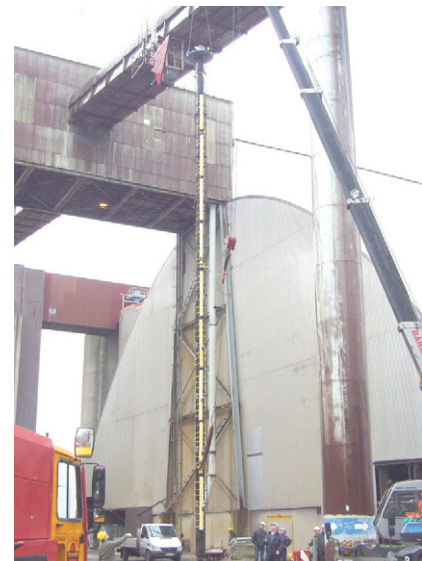
Figure 7. Setting the pump into its vertical position at the terminal.
