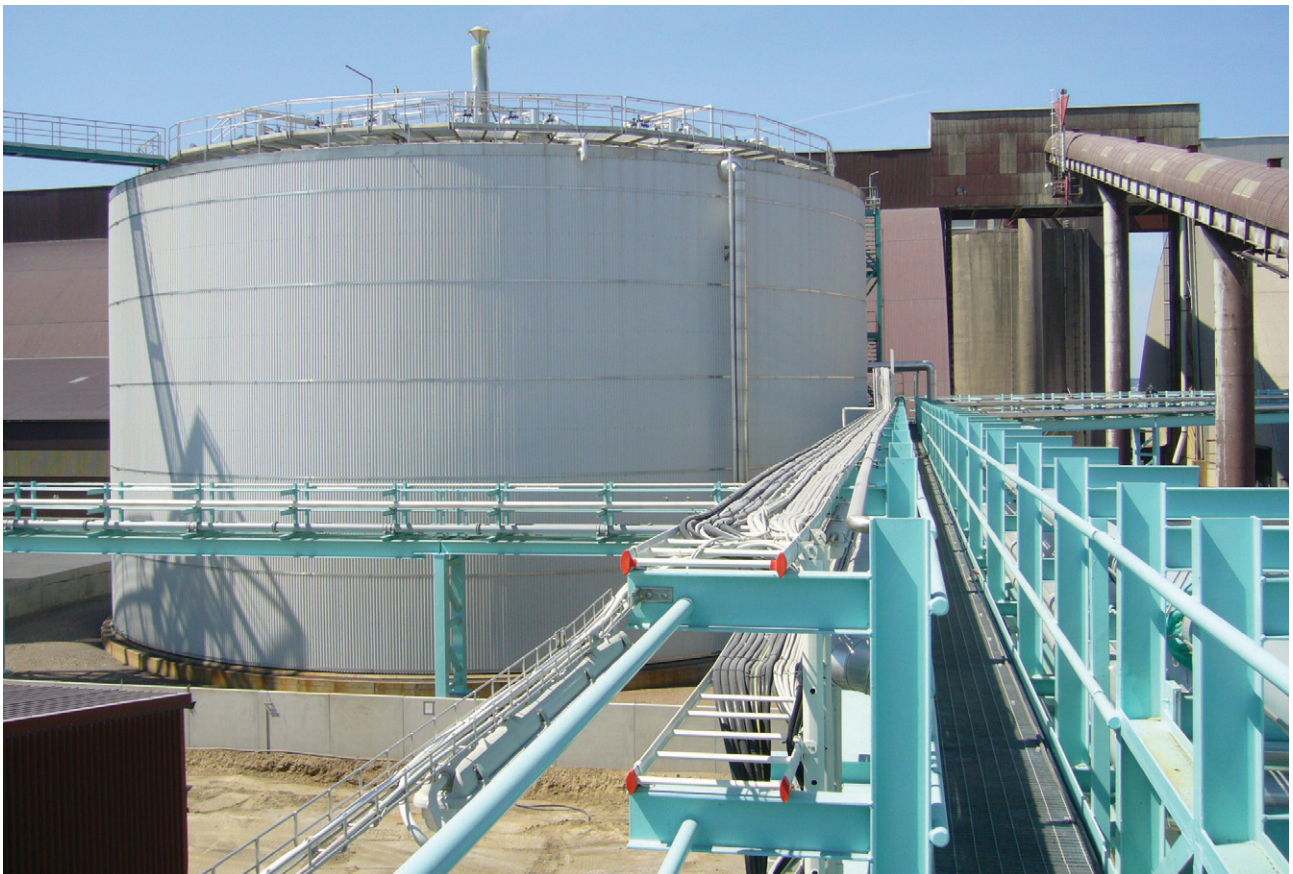
Figure 1. The new sulphur tank installed at the unloading terminal.
